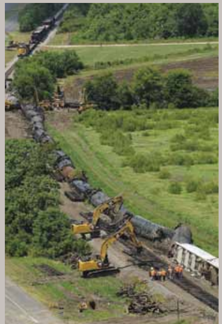
Chemicals leaked from a freight train derailed in Louisiana, US prompting emergency declaration
